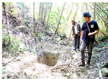
The digging of recharge pits and water collection through rain water harvesting in 2011
