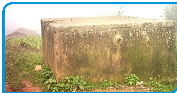
Abandoned water tank, Soi Village, Basar (2008)
