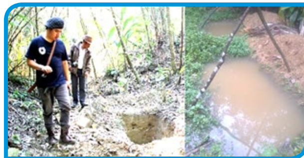
Recharge pit digging and recharge of catchment area
