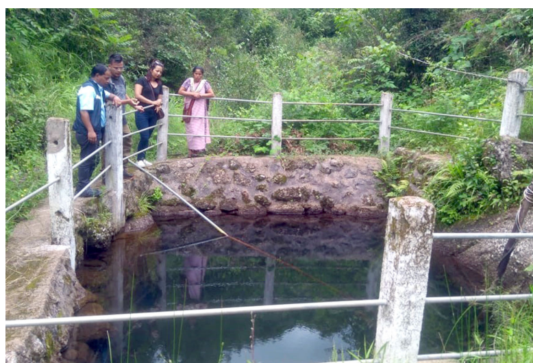
Figure 2. Artificial created reservoir at the lower level of Langlewvillage, Mawthaidraishan, WKH; there is a pipe connected to a generator which pumps out water from this spring tapped chamber to the elevated sections of the nearby villages.
