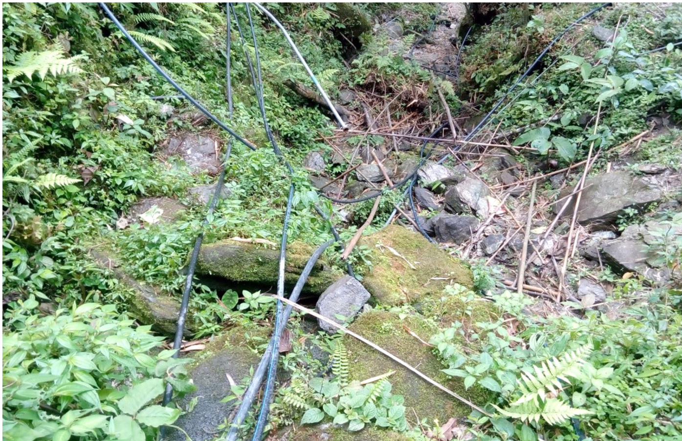
Fig 4: Overtapping around the spring source as seen in Deythang, West Sikkim
