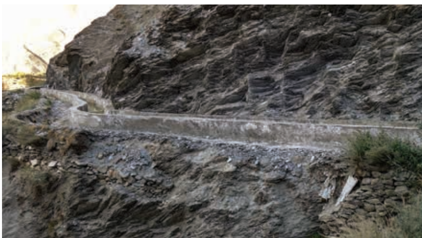
Photo 2: Concretised section of FMIS in 2016 (same section shown in Photo 1)
