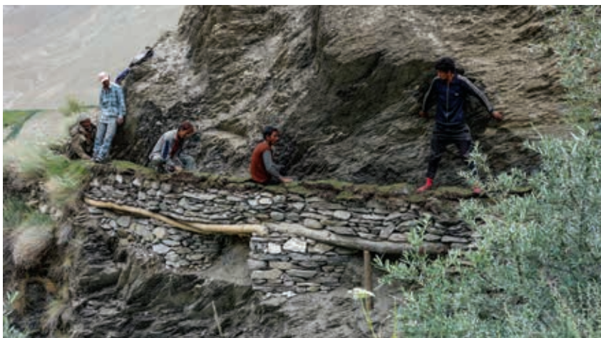
Photo 1: Villagers repair collapsed section of a FMIS in 2013
