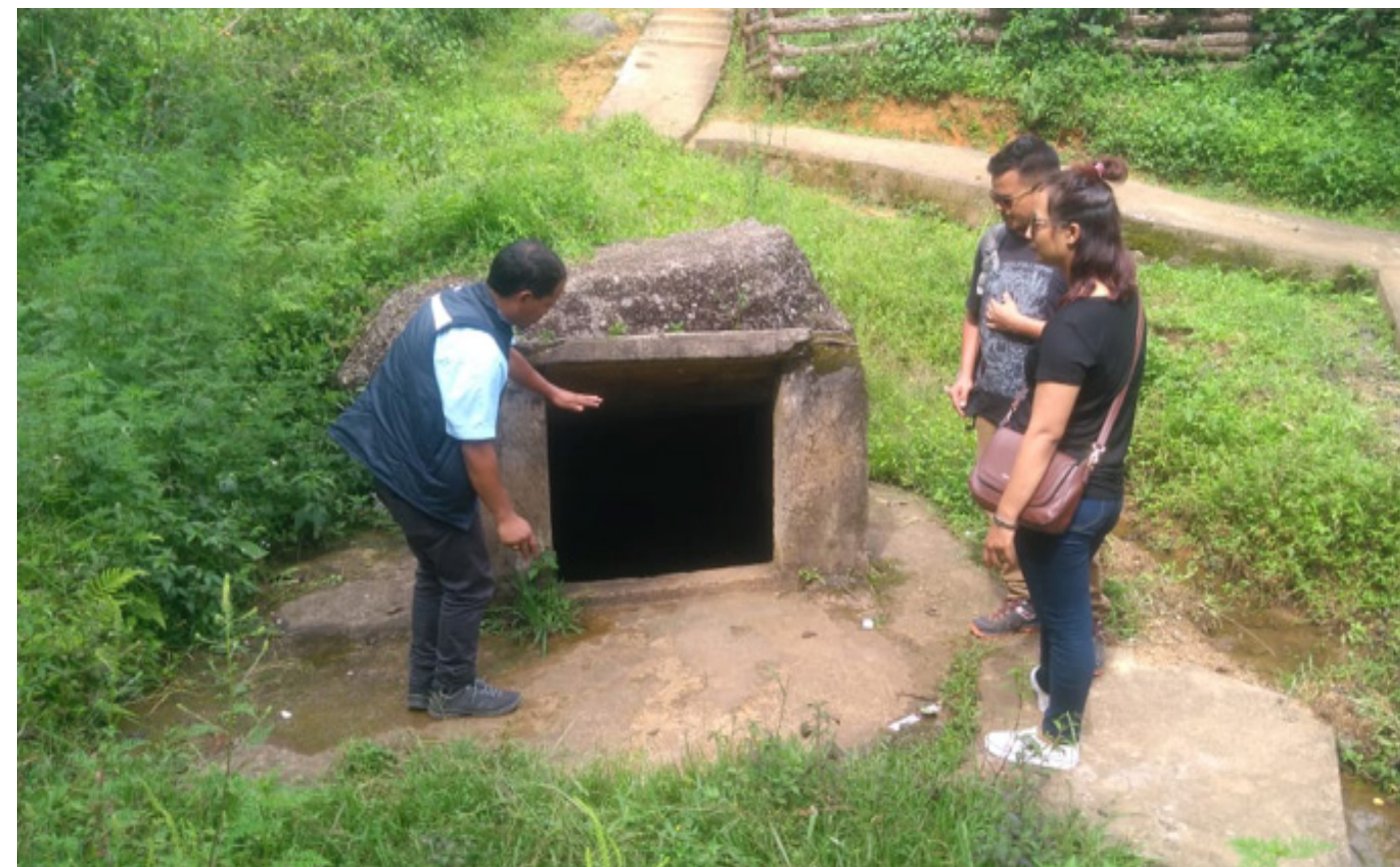
Figure 7: Mr. Bor Borshemlang Saiborne of NERCoRMP explaining how a spring tapped chamber has been constructed to tap the underground springs and help prevent sedimentation making it more hygienic for domestic use.
