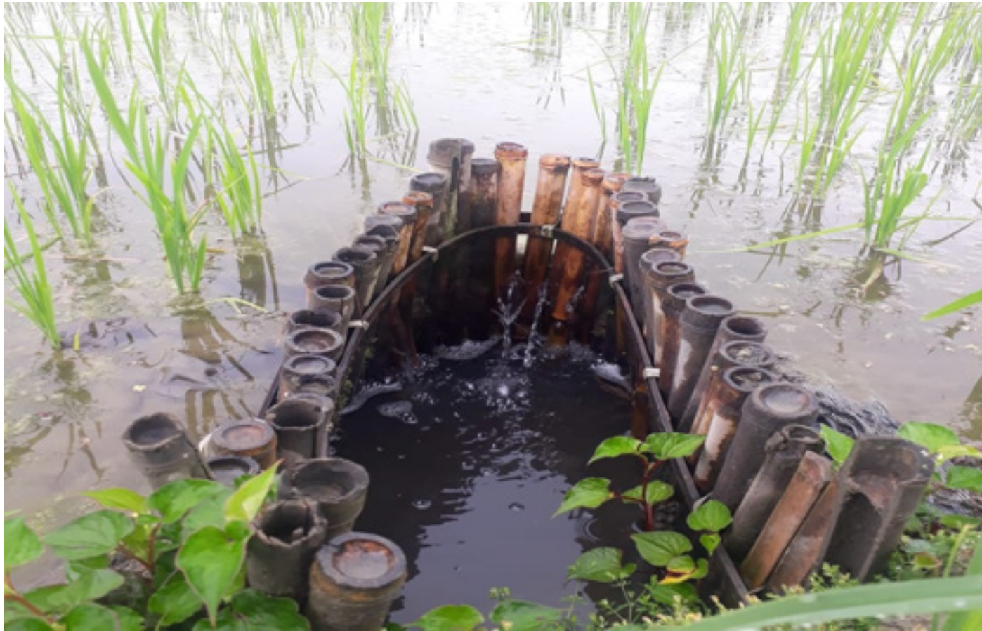
Fig 5: Traditional water supply system(checks water table in the plot and act as supply of water for the adjacent plot)
