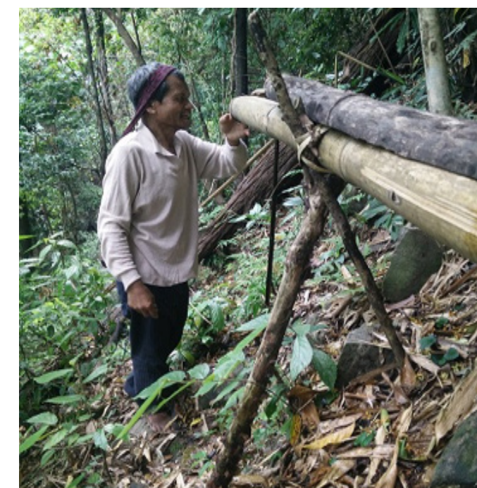
Figure 9: Cultivator indicating how bamboo channels are mounted on Y shaped axis to provide support to the system and tethered with bamboo strings
