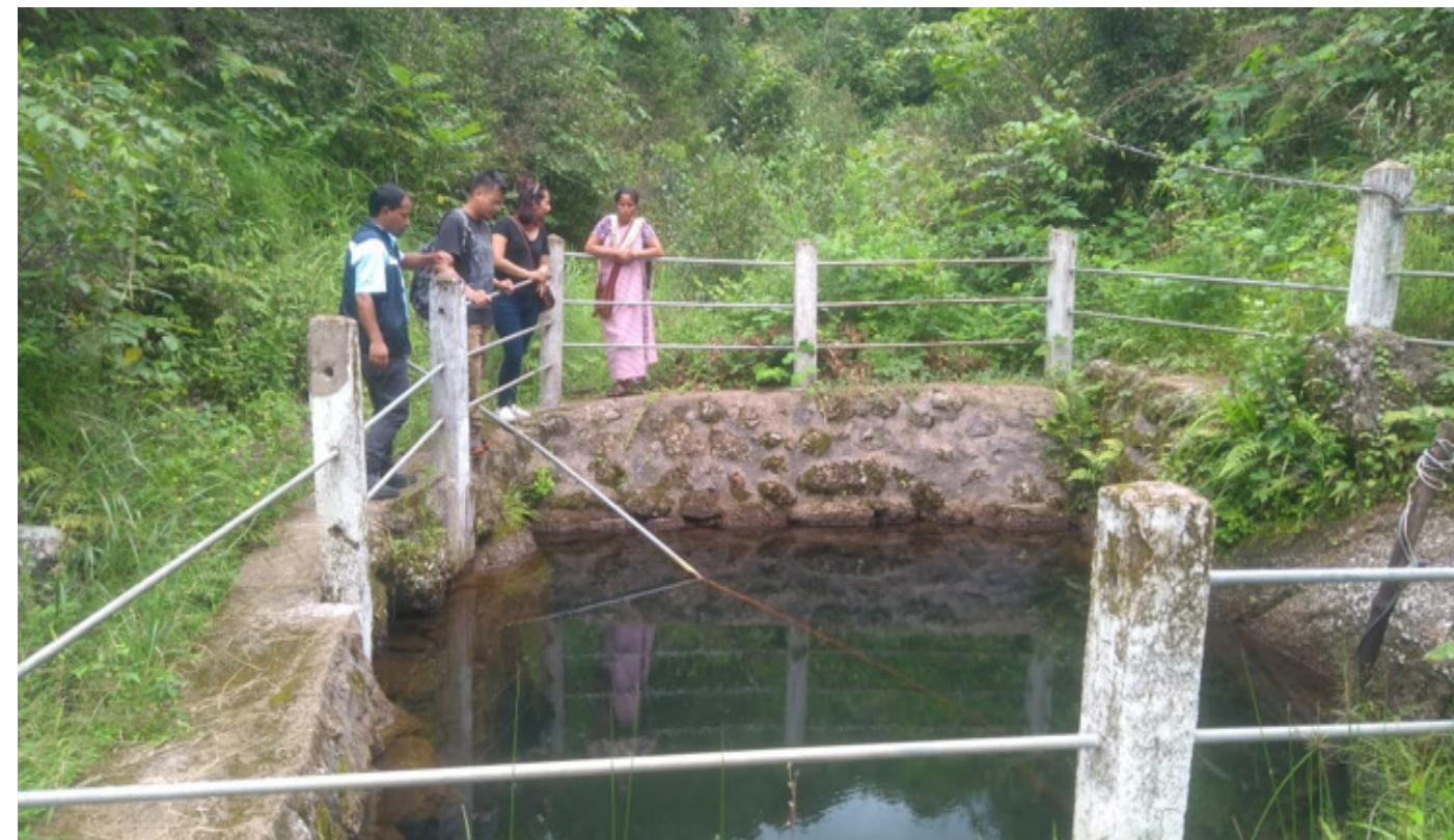
Figure 6: An artificial reservoir at the lower level of Langlew village, Mawthaidraishan, WKH; there is a pipe connected to a generator which pumps out water from this spring tapped chamber to the elevated sections of the nearby villages.
