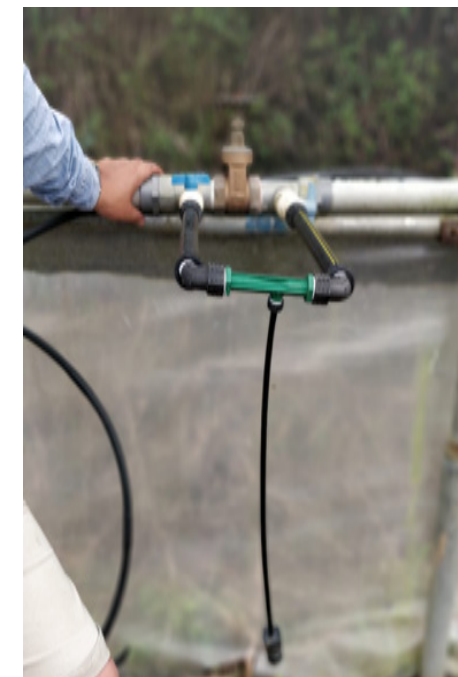
k & l) The above photo plates shows the connection point for the drip line where size of the main line pipe is 40mm and sub main line is 30mm and the size of the lateral pipeline for the water dripped near the plants is 16mm.
